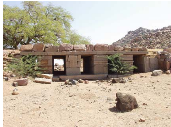
Water Management and Reservoirs in India and Sri Lanka. Fig. 6 Masonry waste weir, or spillway, to regulate high water levels at the edge of a Middle Period reservoir embankment near the village of Kurugodu (photo by Kathleen D. Morrison).
